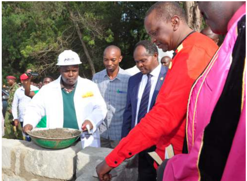
President Uhuru Kenyatta lays the foundation stone for the construction of Koitalel Samoei University College. Looking on is the Vice Chancellor, Prof. Peter Mbithi
